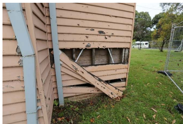
Figure 45. Damage to cladding at south-eastern corner.
