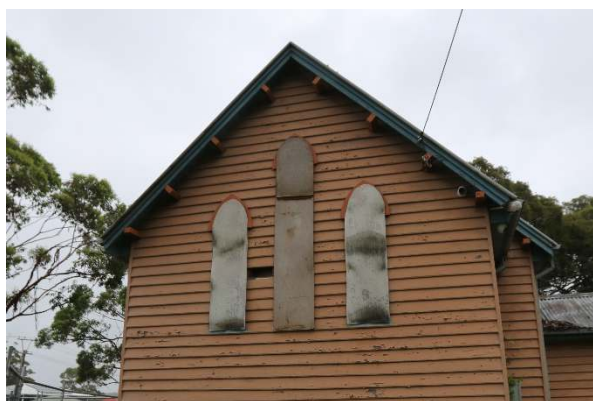
Figure 44. Damaged cladding to eastern elevation.
